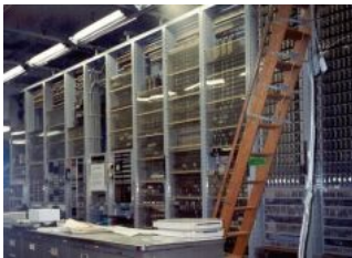
Master Test Frame for #5 Crossbar Switch
