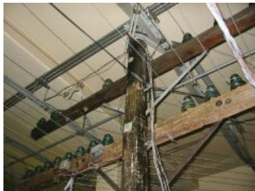
Open wire lead is composed of telephone poles, crossarms, insulators and wire which are visible in this photograph.
