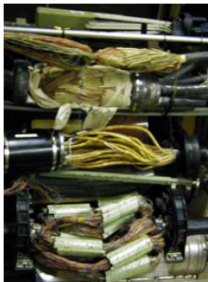
Splices shown are a fiber optic splice, early paper and paper pulp splice, and cable splices.
